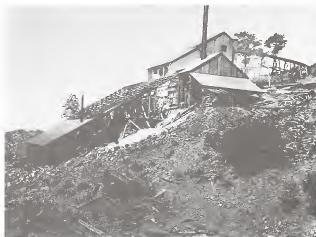
Figure 7. The Exposed Reef Mining Company constructed this 40-stamp processing mill around 1901. Photo courtesy Arizona Historical Society (AHS #72808).
